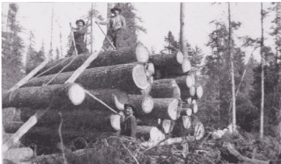
Fig. 11. Decking Logs on Skidway.
