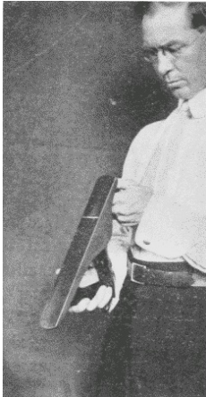
Fig. 102. Sighting Along the Sole of Jack-Plane.
