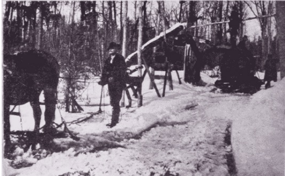
Fig. 10. Making an Ice Road by Flooding.
